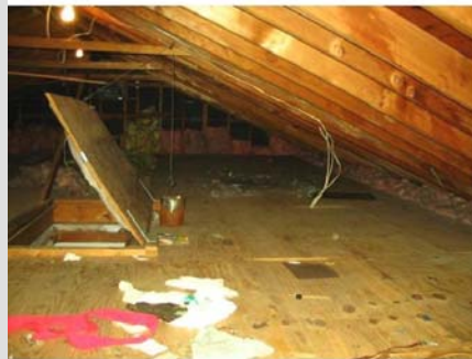
Rear of attic area.
