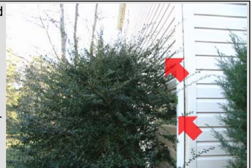
Keep branches trimmed away from structure
